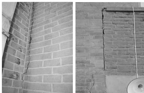
图 9 墙体及搭建房屋与主体结构接缝竖向开裂 Fig.9 Crack of wall and crack between annex with the main structure
