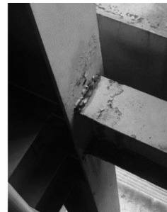
c 焊缝区域涂层优先脱落 [64]
