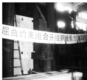
图5 试件安装完毕照片 Fig.5 Specimen S1 Installed
