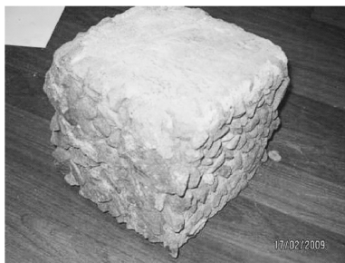
图2 混凝土受酸腐蚀后的外观形态 Fig.2 Degradation of concrete after acid attack
